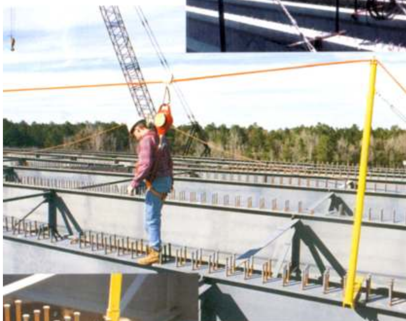
Above: SkyGirder with Permacable in use for bridge construction
