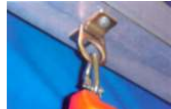
D-Ring Plate • Bolts or welds to anchorage • Reduces the chance of burst-out or roll out • Provides identifiable, permanent fall protection anchorage
