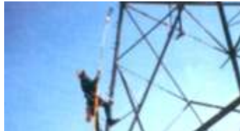
Ankalok - Extension Pole Anchorage • First man up anchorage connector • Fiberglass "hot stick" pole extends up to 24 feet • Available with several fall protection systems
